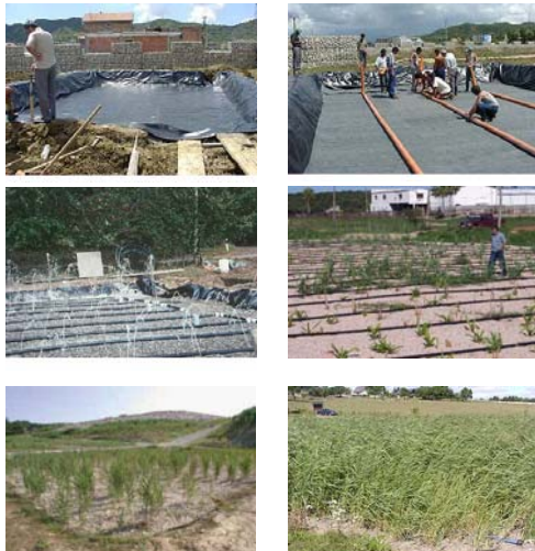
Pictures: Setting up and building constructed wetlands can be done using local workforce and material.
