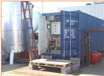
Picture: Container with 10m 3 locally produced warm water storage tank 80°C, for 22 hour water production
