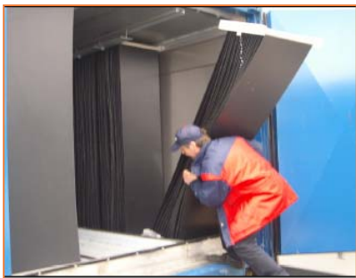
Picture: Condensation within the container
