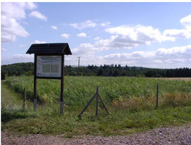
Constructed wetland currently: Front view
