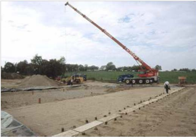
Construction during September/October 2001 – 2 months only
