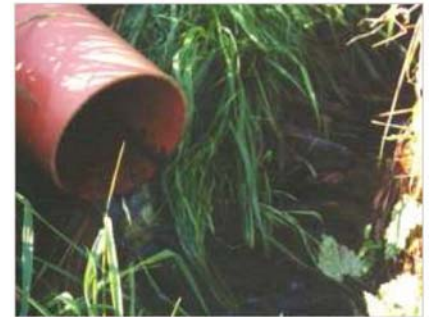
Clear water leaving the constructed wetland and feeds the nearby river
