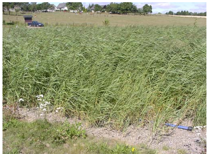
Constructed wetland currently: rear view with homes on the top
